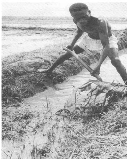
Fig. 15 Construction of an earthen canal
